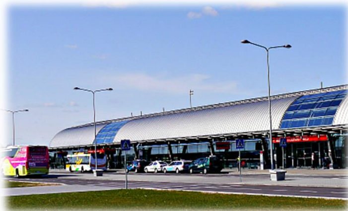
Modlin airport, Warsaw
